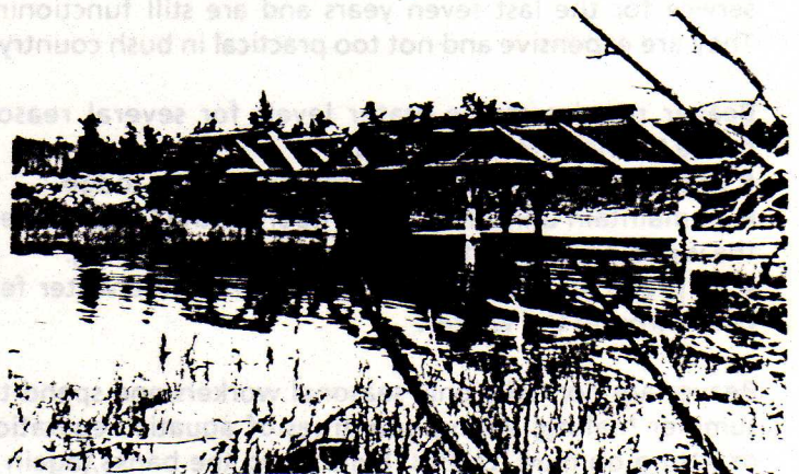
Wood bridge over Beaver Creek -(remnants of wood pilings still visible)
